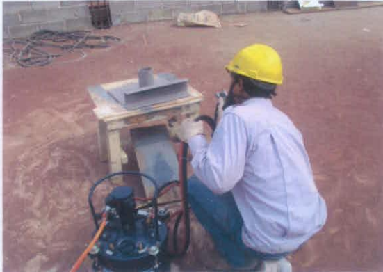
IN PROGRESS BLASTING PAINTING
